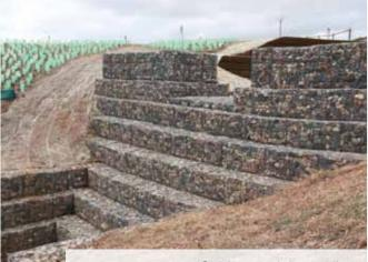
Gabion retaining walls
